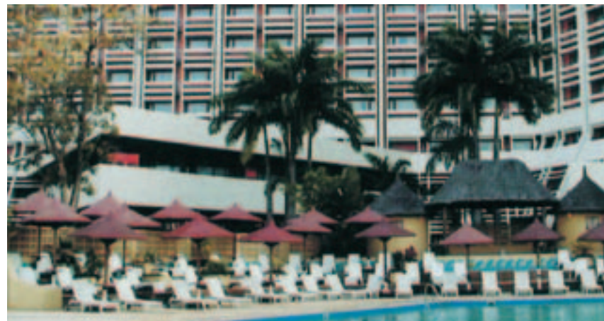
The Nicon Hilton in Abuja has been undergoing a $40 million (£22 million) upgrade.
